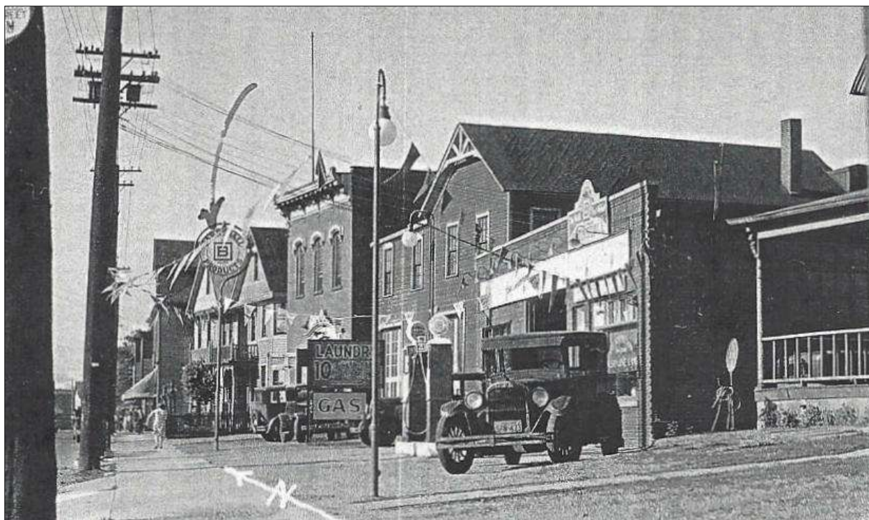
Figure 12. View of Scranton Road, north end, facing northeast including Cleveland Fire Engine Company #8 and Home Family Laundry & Gas Station, Photo 1933
