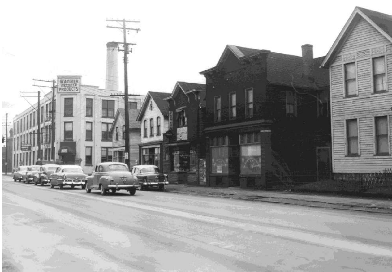
Figure 11. Wagner Awning Building, Starkweather Business District, Photo 1954.
