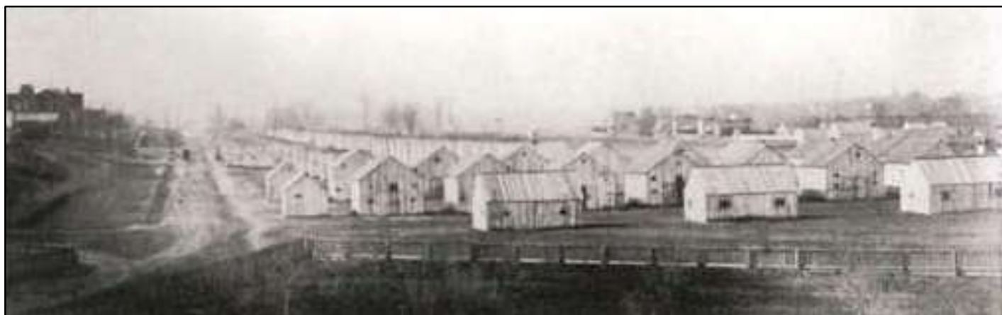
Figure 7: Barracks buildings at Camp Cleveland, most likely viewed from the intersection of what is now West 7 th Street and Marquardt Avenue looking north. Note Cleveland Institute (erected in the 1850s as part of the short-lived Cleveland University) at far left.
